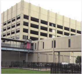
Gravier St. parking garage and Walkway
